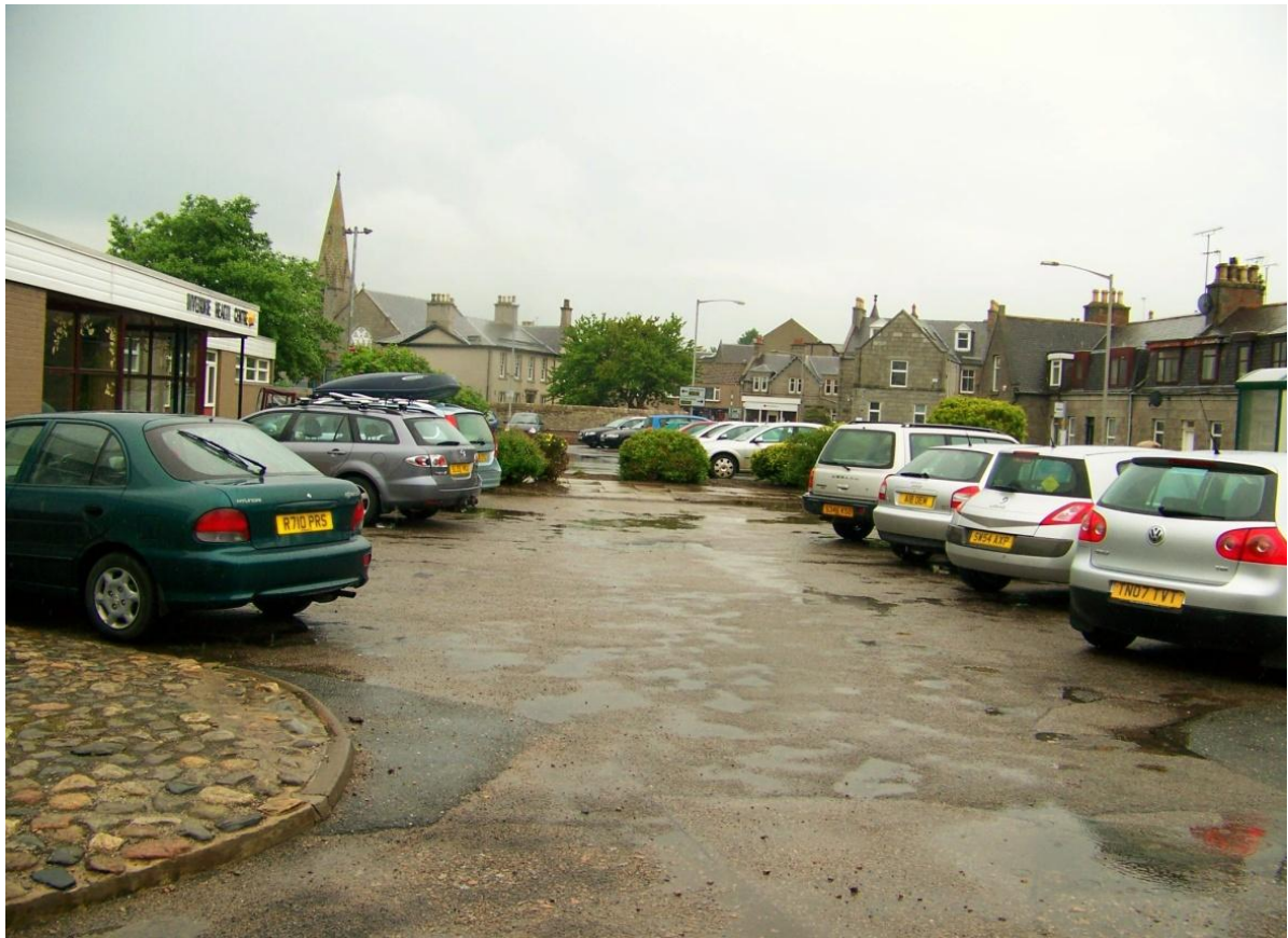
Fig 7: Inverurie External- Overcrowded Car Park. Liable To Pot Holes and Flooding
