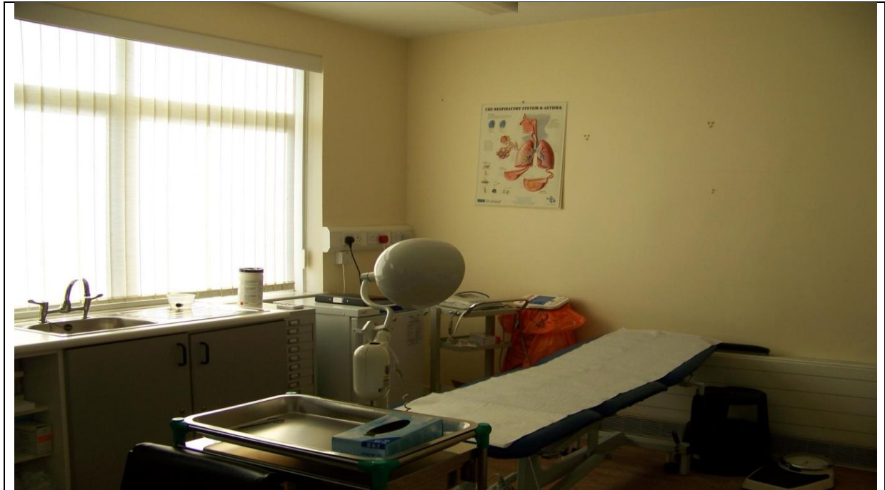
Figure 5: Pictures of the Internal and External Building Condition at the Northfield Surgery.
