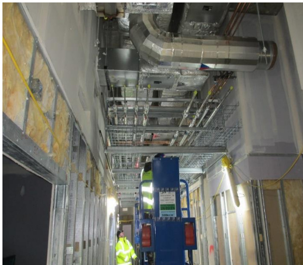
The Baird Family Hospital - Ground floor corridor, pipework module installation ongoing.
