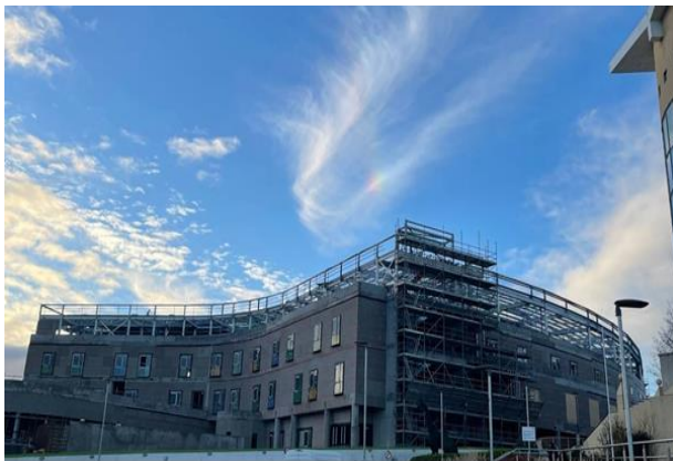
The Baird Family Hospital East Side – curtain walling in progress
