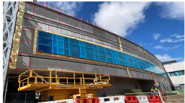
East elevation ready for external render work
