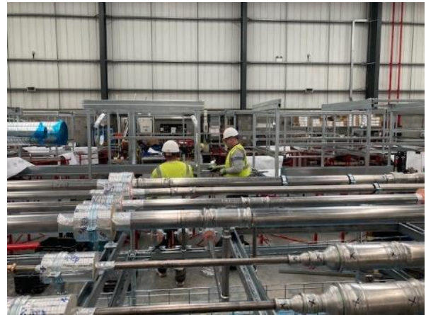
Factory visit to inspect services modules
