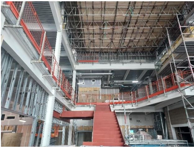
The ANCHOR Centre feature staircase
