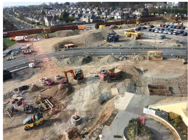
Ongoing building work on the Baird site and RACH car park.
