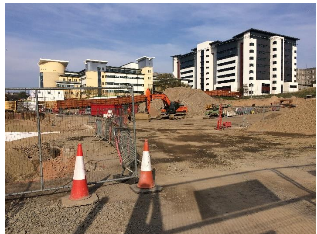
The ANCHOR site preparation in progress.
